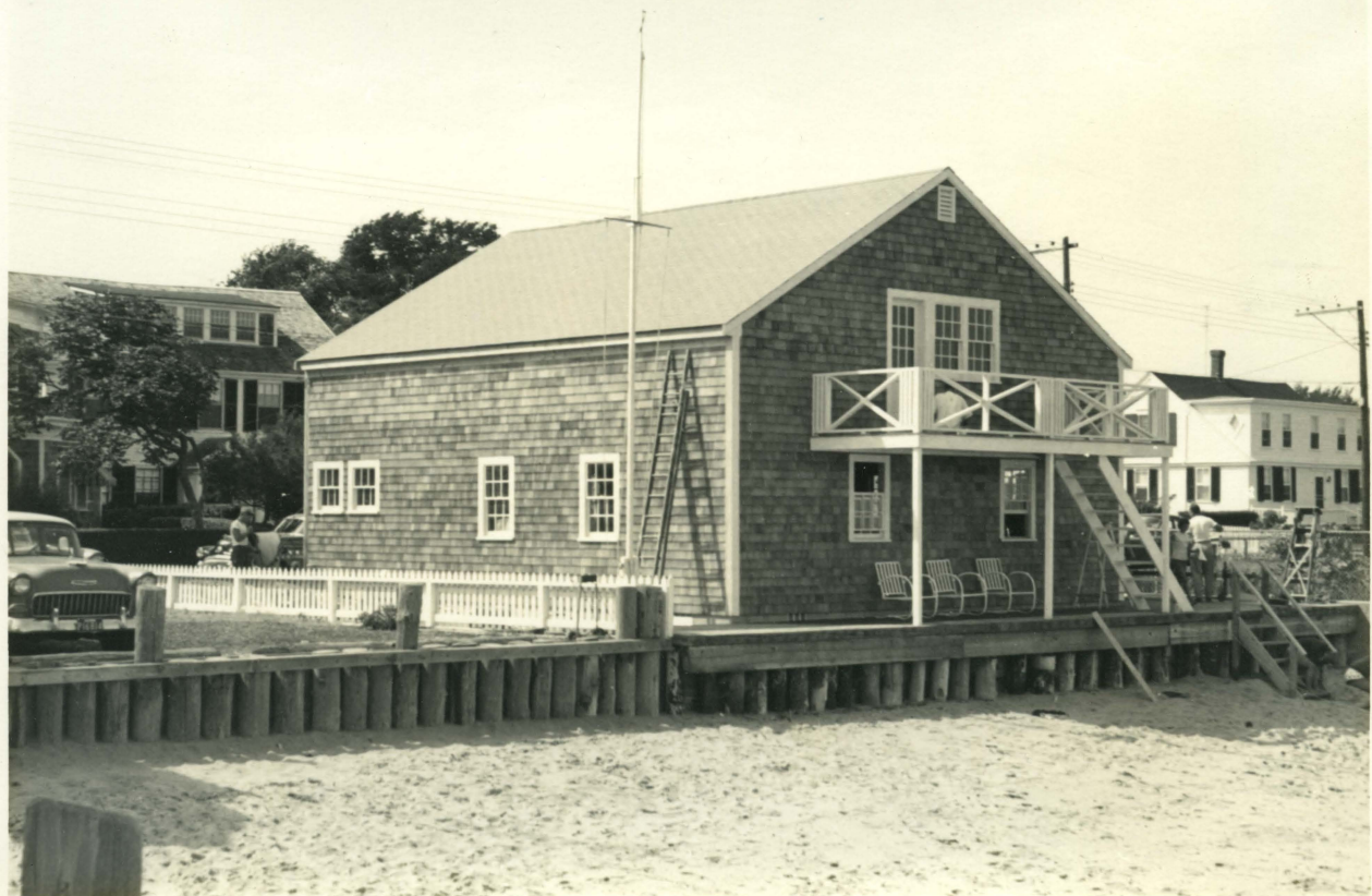
West End Racing Club - 1950's Construction nearly finished
