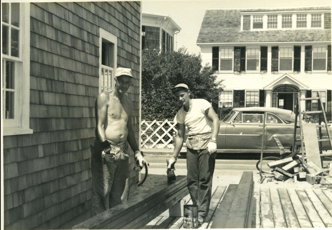
West End Racing Club - 1950's Painters sealing the deck timbers Hans Hoffman house in the background
