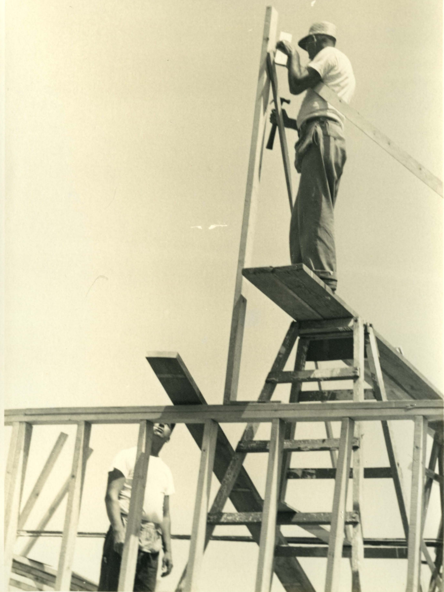
Roof construction on the West End Racing Club - 1950's
