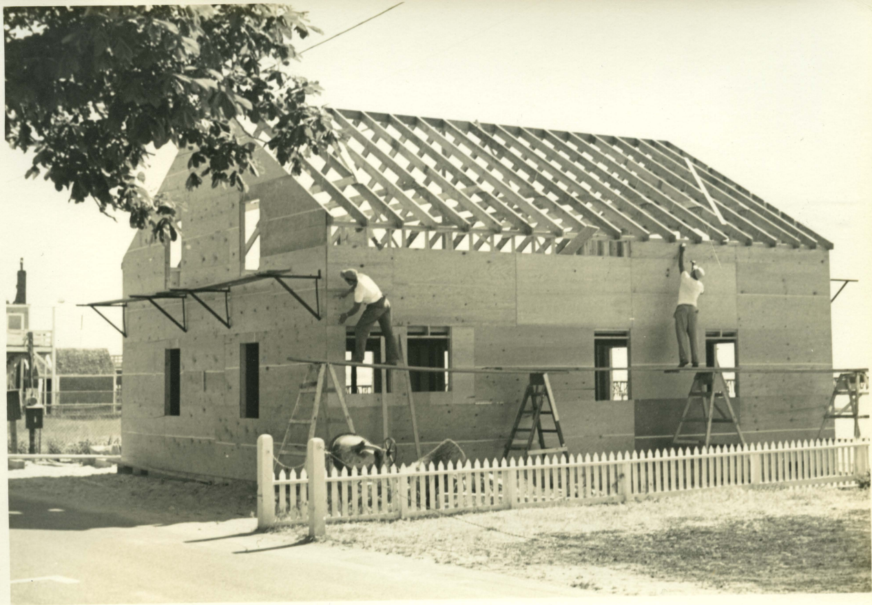
Roof rafters in place on the West End Racing Club - 1950's
