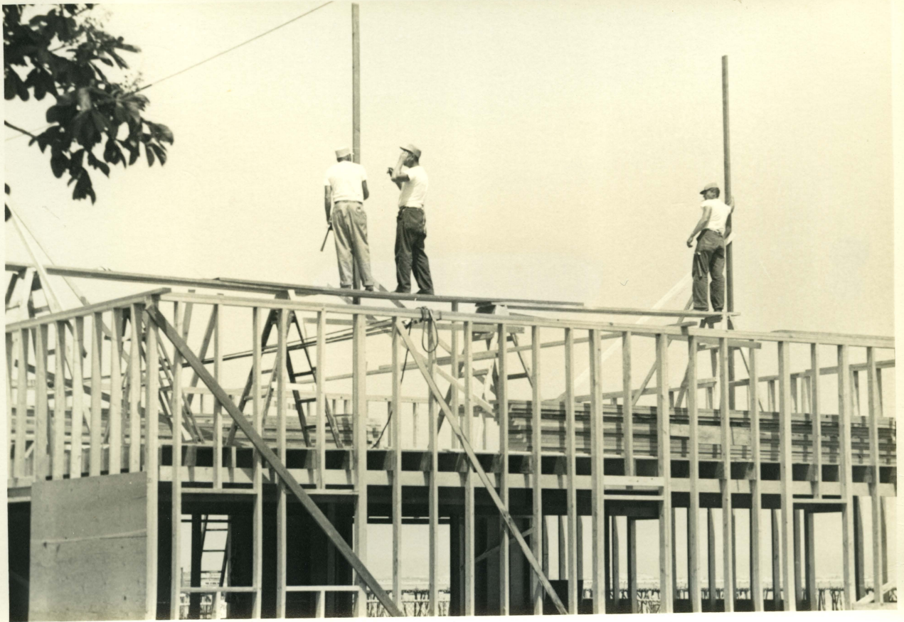
Getting ready to raise the roof of the West End Racing Club
