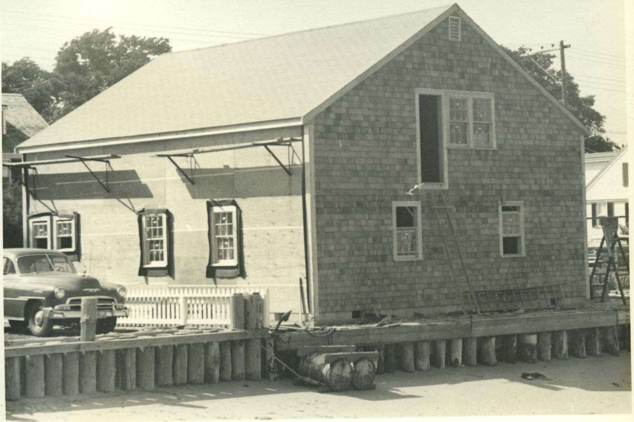
West End Racing Club under construction - 1950's windows are in, roof is on
