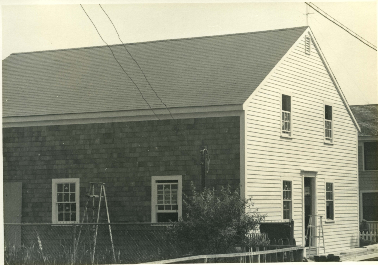
West End Racing Club - 83 Commercial Street construction is nearly finished - 1950's
